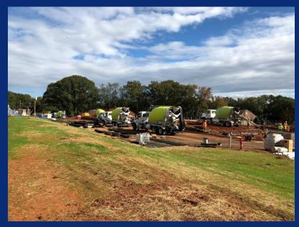
Concrete truck convoy on site for braced frame foundations
