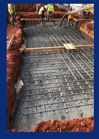
Braced frame foundation being poured
